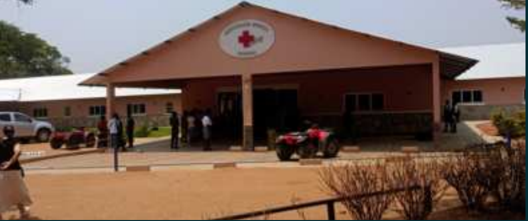
New entrance & ward at Chitokoloki Mission Hospital
